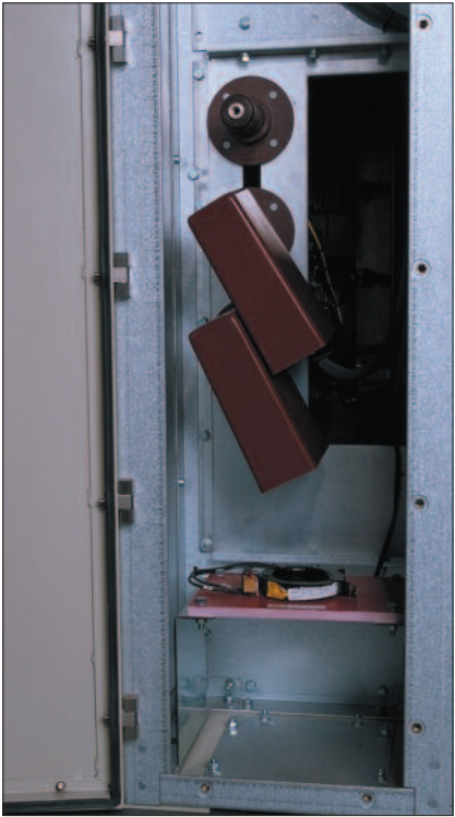
VCU Cable Termination Compartment c/w Optional CBCT
